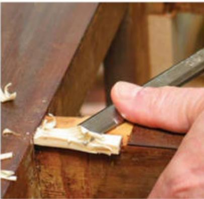
**Trim the patch.** The patch should be left proud, then trimmed level with the substrate.
