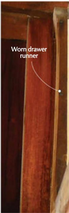
**Worn drawer runner.** Drawer runners, the strips of wood that drawers slide on, typically become hollowed out after many years of use. They should be replaced.
