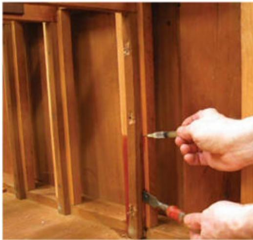
**Remove the runners.** The runners in this chest-of-drawers were nailed and glued with animal hide glue. They were easy to remove by first removing the nails, then crystallizing the glue bond by inserting denatured alcohol. Finally, applying pressure with a chisel separated the bond.
