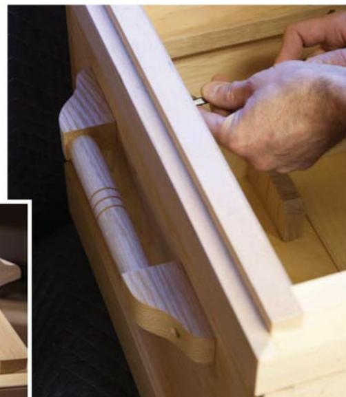
**Screwed either way.** Affix the lifts with stout #8 screws from both the inside and outside of the carcass.
