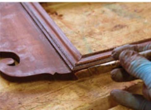
**Matte it down.** Using an artist's brush, coat the sanded surface with matte shellac. As the alcohol evaporates, you will see the sheen dull in only a minute or two.
