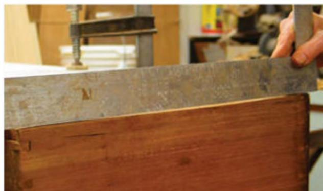
**Worn drawer sides.** Like the runners, the bottoms of the drawer sides also wear concave after many years of the drawers sliding in and out of a chest.
